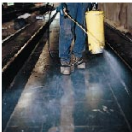
Spray application of DMA 2000 FORM-RELEASE AGENT
