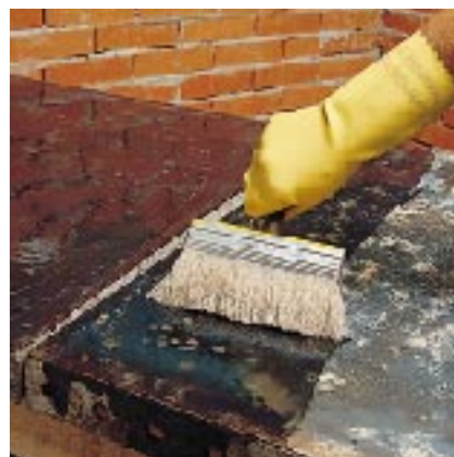
Applying DMA 2000 FORM-RELEASE AGENT with brush
