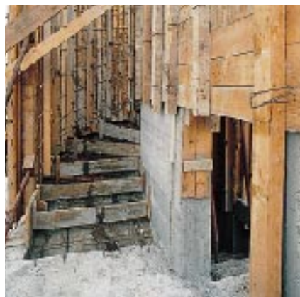
Examples of formwork treated with DMA FORM-RELEASE AGENT
